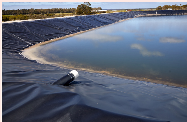
Secondary liquid effluent storage pond.
