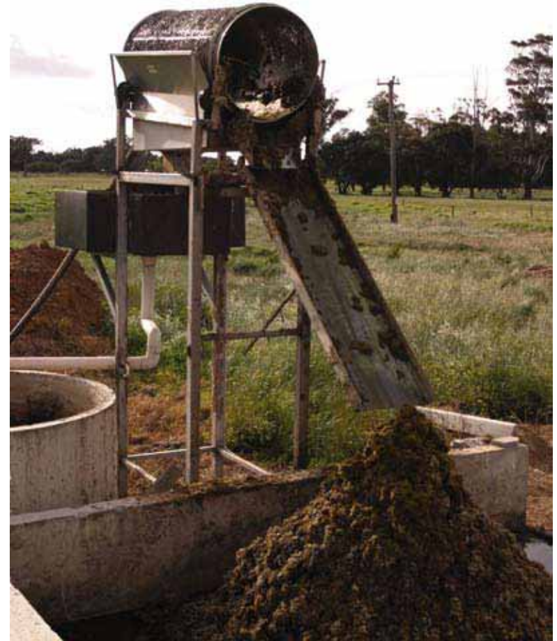
Solid effluent separation systems like the one above provide a source of organic material that can be added to the soil to improve soil structure.
