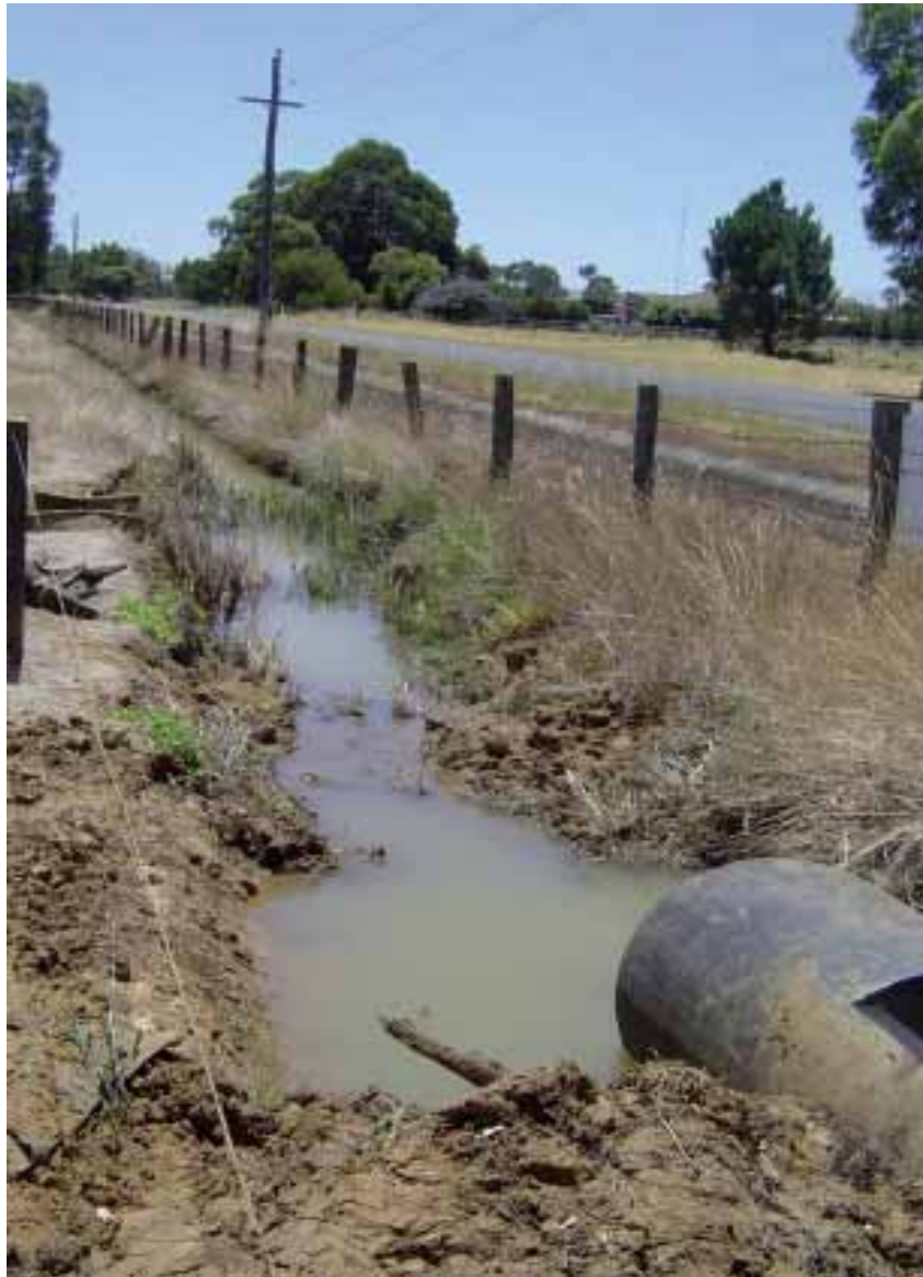
Head irrigation ditch at the Hanks Dairy in Harvey
