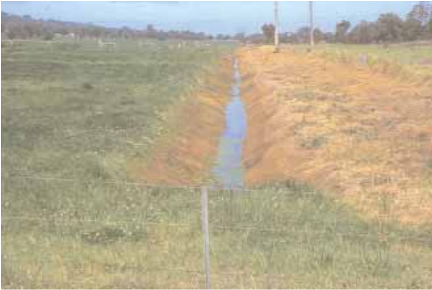
FIGURE 5.8 Flood irrigation surface drain.
