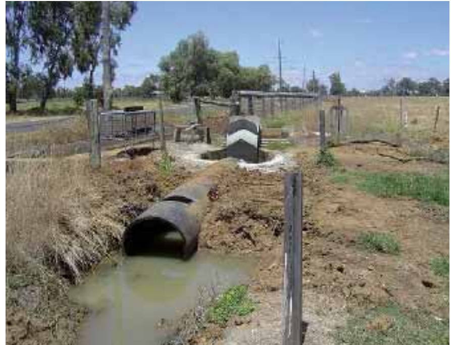
Dethridge wheel at the Hanks Dairy in Harvey
