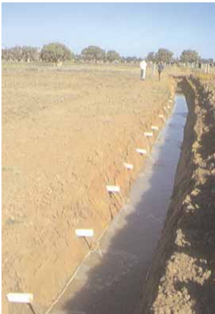
FIGURE 5.7 Subsurface pipe drains.
