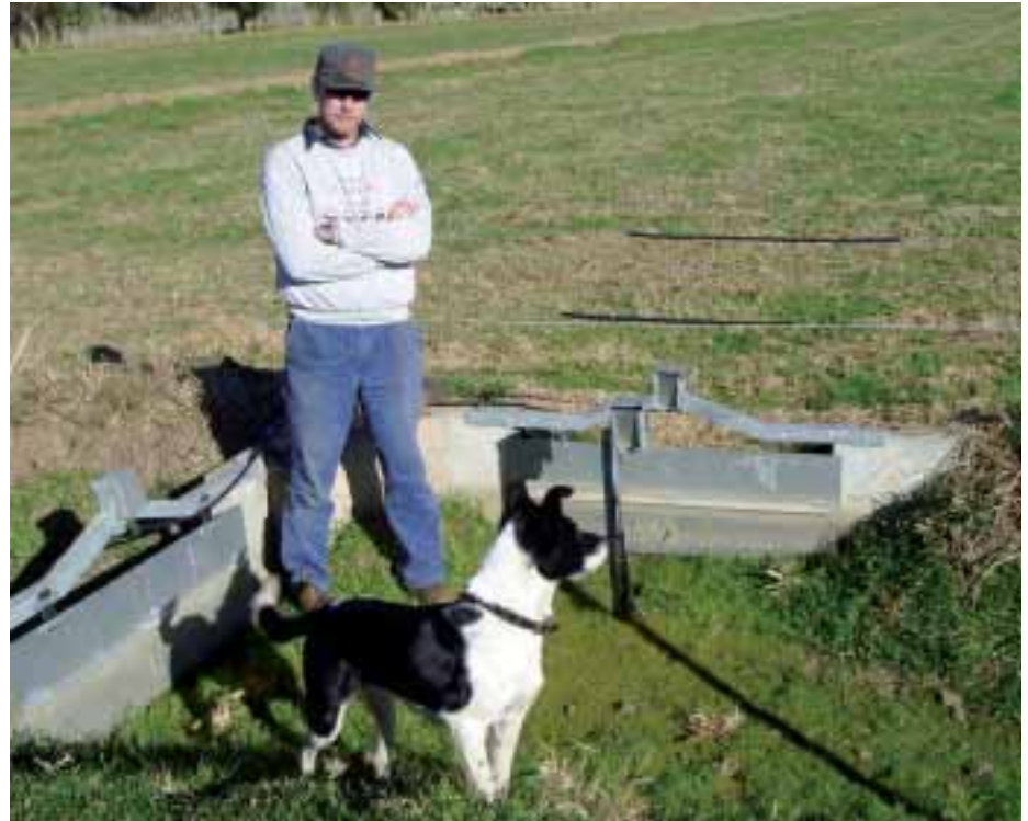
Automated flood gates installed on the Depiazzi farm
