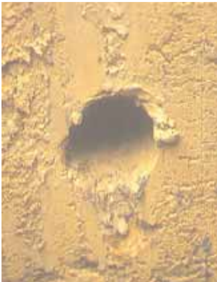
FIGURE 5.9 Mole drain
