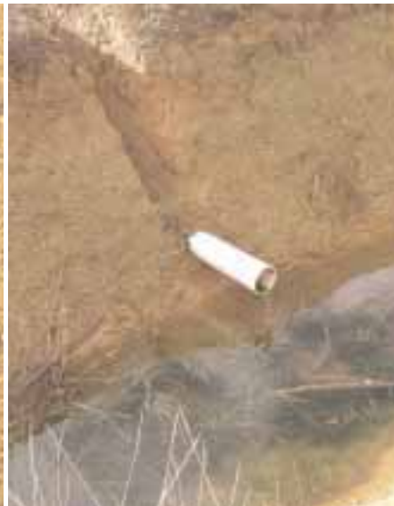
FIGURE 5.10 Buried pipe drain
