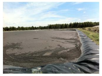
Figure 2 Uncovered Anaerobic Lagoon (Juice factory)
