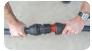
7. It is important the fitting is assembled in the correct order (above). Push both ends of the O-Ring into the threaded joint, ensuring O-ring sits firmly and is not twisted or rolled as this is crucial to the integrity of the joint.
