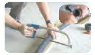
2. & 3. The two most common methods of cutting pipe is with a hacksaw or using pipe cutters. It is important to cut the pipe squarely. If joining two lengths of pipe, ensure the ends are also square.
