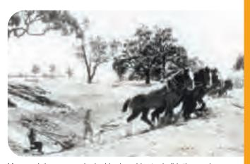
Men and horses worked side by side to build the early channels and dams. Over time, this gravity-fed system expanded to include 12 storages that divert water from the Wimmera and Glenelg rivers and various lakes. More than 17,500km of open earthen channels deliver water from these storages to over 20,000 dams.
