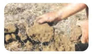
Soil types and condition impact on the quality of pipe installation. Sometimes the pipe route needs to be pre-ripped a number of times. This may result in large clods rising to the surface. It is good practice to breakdown the clods by running machinery wheels over them before the final pass of inserting the pipe.
