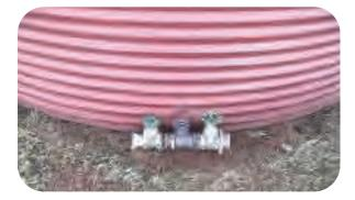
A spray cart fitting can be installed on one connection and a CFA fitting on the other (above).
