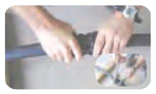
8. Hand tighten the locking collars over the threaded joint before using two pipe wrenches or multigrips (inset) to tighten the joint.
