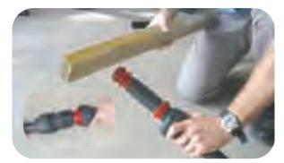
6. Place the threaded collar and tapered locking ring on the pipe before pushing the O-ring insert into place. These inserts not only have a barbed profile but are also slightly tapered to ensure a tight fit. The rings also have internal barbs to ensure the pipe cannot slip out.
