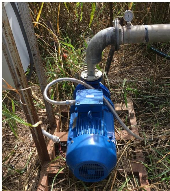
The energy used per ML pumped per metre of Total Dynamic Head is used to compare the performance of pumps with different duties. In 2016, when supplying the 'Hill' pivot, this measure was 6.7 kWh/ML/m and when supplying the 'Flats' pivot it was a whopping 25.7 kWh/ML/m, both in excess of the accepted benchmark of 4 kWh/ML/m.
