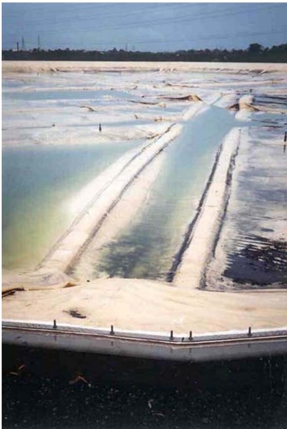
Figure 19 Negative Pressure Covers for Anaerobic Lagoons (Poultry Processing CAL)
