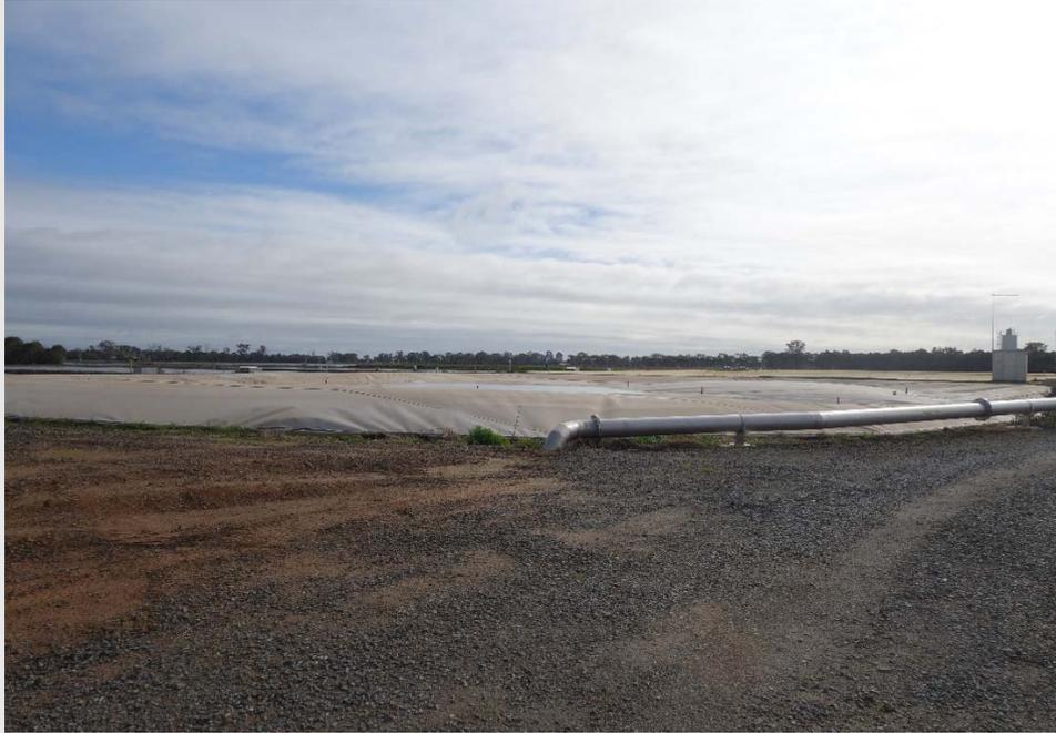
**Biogas collection pipework (from above ground to underground to knock out pot)**
