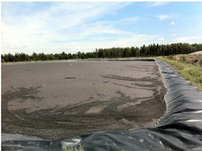
Figure 2 Uncovered Anaerobic Lagoon (Juice factory)
