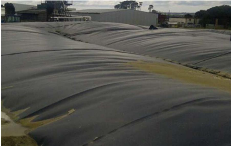
Figure 18 Positive Pressure Covers for Anaerobic Lagoons (King Island Meat Processing CAL)
