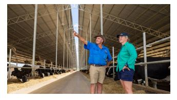
The 2.5m eaves are designed to stop 85 per cent of rain coming in. The large box gutter (300mm x 300mm) running along each side of the shed with only one down pipe at the end. The box gutter is designed to cope with rainfall rate up to 100mm/hr, well above the maximum rate expected for this region.
