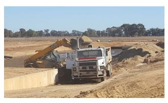
Due to a delay in fitting the screen in the manure solid/liquid separator, slurry filled the first two separation ponds during the initial weeks of operation and had to be removed. However, the separator is now functioning as intended, producing a stream of pressed manure fibre with a dry matter content of 30 per cent. This fibre is conveyed up a belt and deposited on top of a stack. Periodically, it is then removed from the stack and spread over the paddocks as fertiliser.
