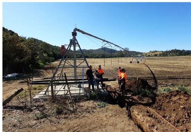
Instalment of a new filter for effluent pumping system
