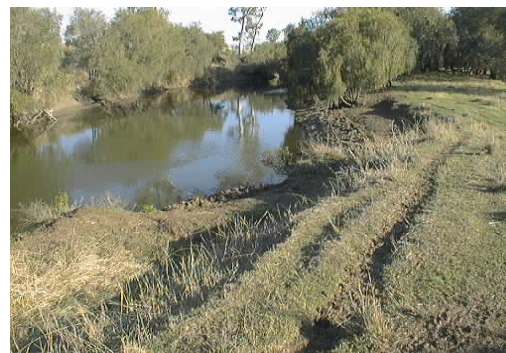
No continuity in woody vegetation. This has contributed to an unstable and widening stream channel.
