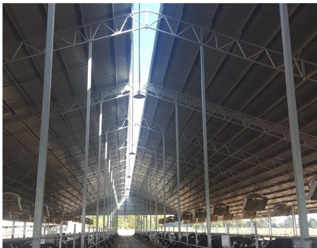
Lights are fitted down the centre of the shed. They turn on at 2:30am to wake up the three-times group of cows prior to milking at 3:15am and switch off again at sunrise when the light intensity in the shed rises above 50 lux. If the light intensity in the shed falls below 250 lux at any time during the day, the lights will turn on. In the evening the lights turn on at about 6:30pm and stay on until 10:00pm.
