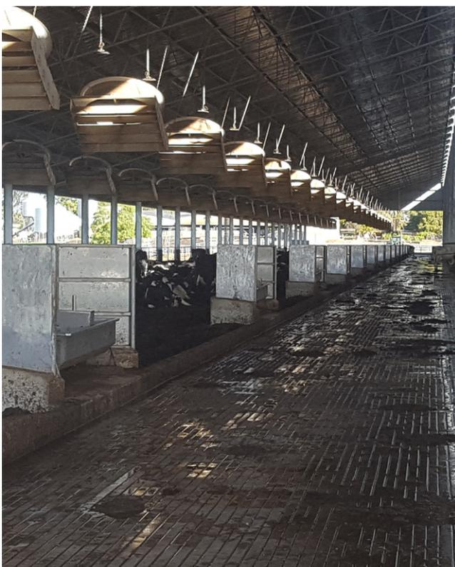
Each tipping metal water trough is surrounded on three sides with a 1.6m high solid metal shield, so that it is only accessible from the cow alley and cows cannot splash water onto the bedding pack. The source used to supply stock water is untreated irrigation channel water. All water troughs are tipped every day to ensure water is fresh and they are cleaned once per week.
