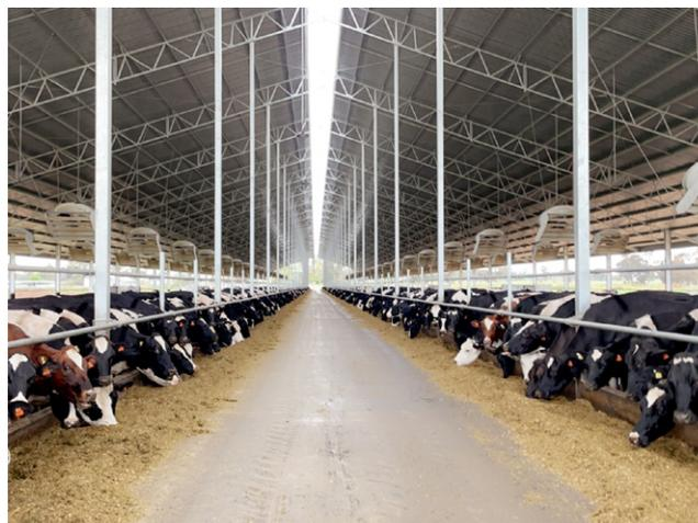
The 2.5m eaves are designed to stop 85 per cent of rain coming in. The large box gutter (300mm x 300mm) running along each side of the shed with only one down pipe at the end. The box gutter is designed to cope with rainfall rate up to 100mm/hr, well above the maximum rate expected for this region.
