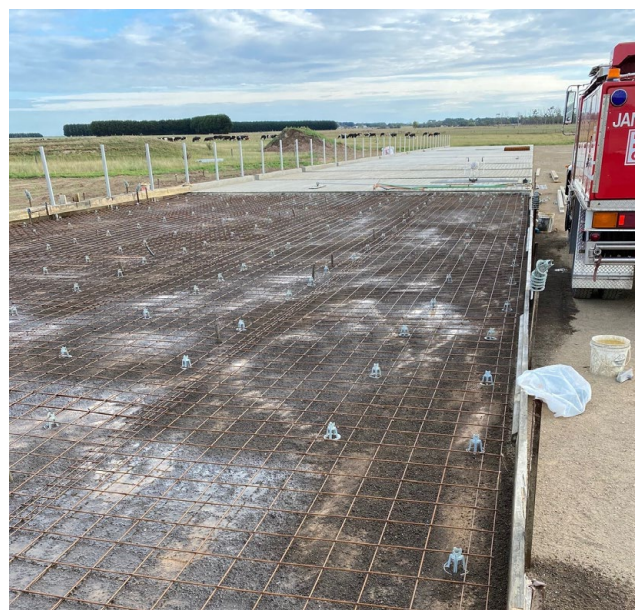
Construction phase of the feedpad.
