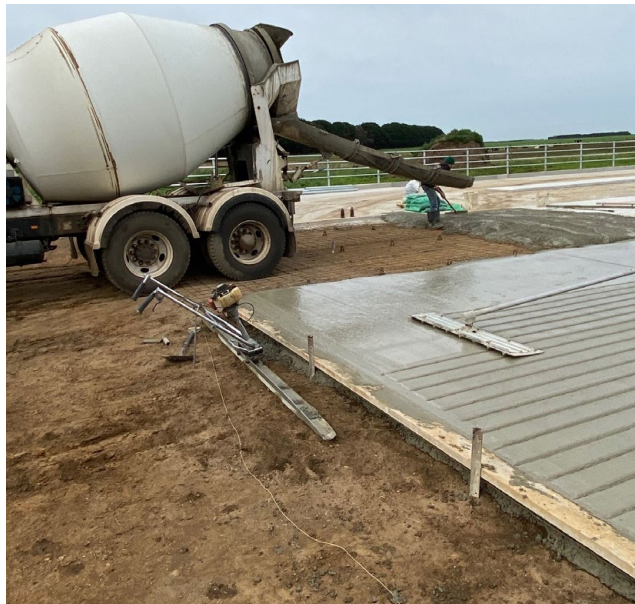
Construction phase of the feedpad.
