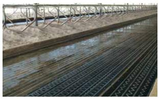
Sand bedded cubicles. Flood-washed cow alley
