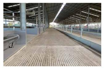
Note: Grooves cut into the concrete in the direction of the alley.
