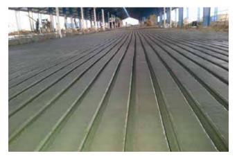
Figure 70. V-shaped groove patterns should be avoided as they result in more slips and an increase in lameness
