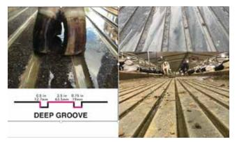
Figure 69. Grooves made by a bull float will never provide as sharp of an edge
