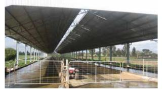
Fully concreted feedpad with nib wall, central feed alley, solid roof and flood wash system
