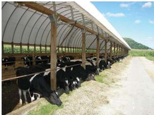
Figure 8. Composting barn with external feed-bunk and curtain.
