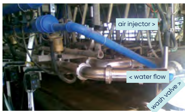
Figure 10 Air injector and wash valve on a looped milk line (example only)
