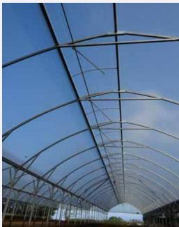
Vents in the roof can be manually or automatically opened to allow hot air to escape when necessary.
